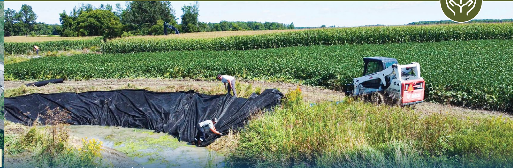
Erosion control project in South Glengarry.
